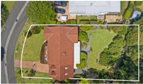
5 O'Connell Place, Gerringong
