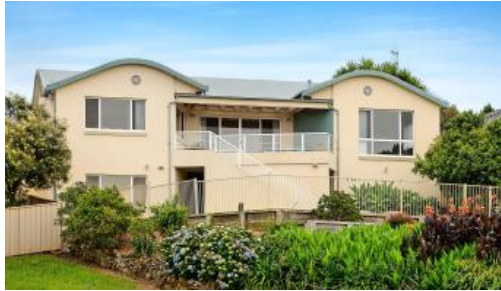
13 Coolangatta Avenue, Gerringong
